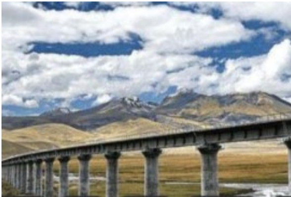
Sichuan-Tibet Railway Construction
