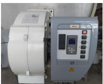
Boiler low-nitrogen burner transformation
