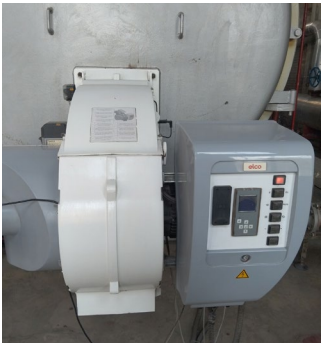
Boiler low-nitrogen burner transformation
