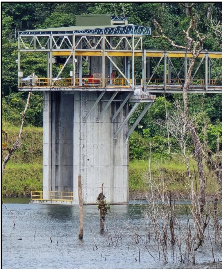
Figure 2: Spillway Tower at the Cobre Panama TMF
